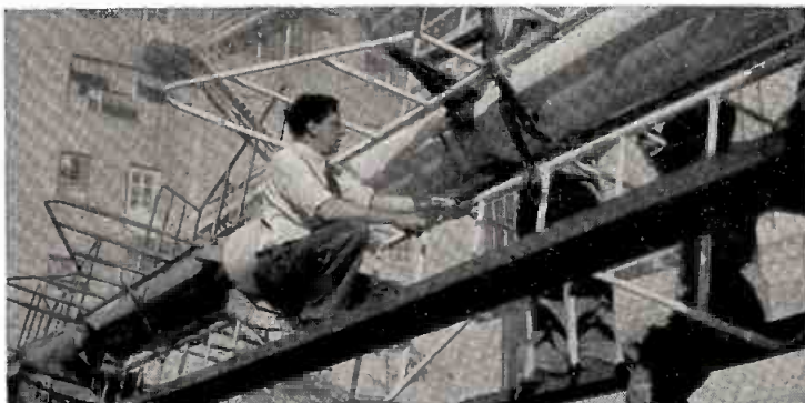
Clem Castle, Storer Broadcast Company engineer, inspects the General Electric 6-Bay Antenna before hoisting to the tower.
